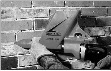
PHOTO: SPEC-JOINT 46 can be used in electric pointing guns without special admixtures or mix modification.
